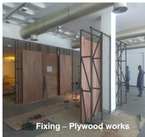
Fixing - Rectangular tubes
