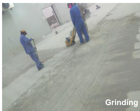
Concrete Smooth finishing
