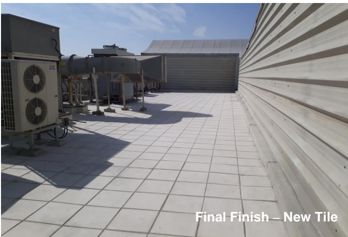
Roof Floor Tiles Gap Filling by Sand
